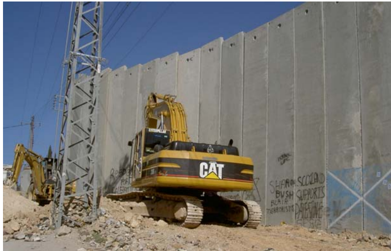
The wall under construction in Abu Dis, East Jerusalem
